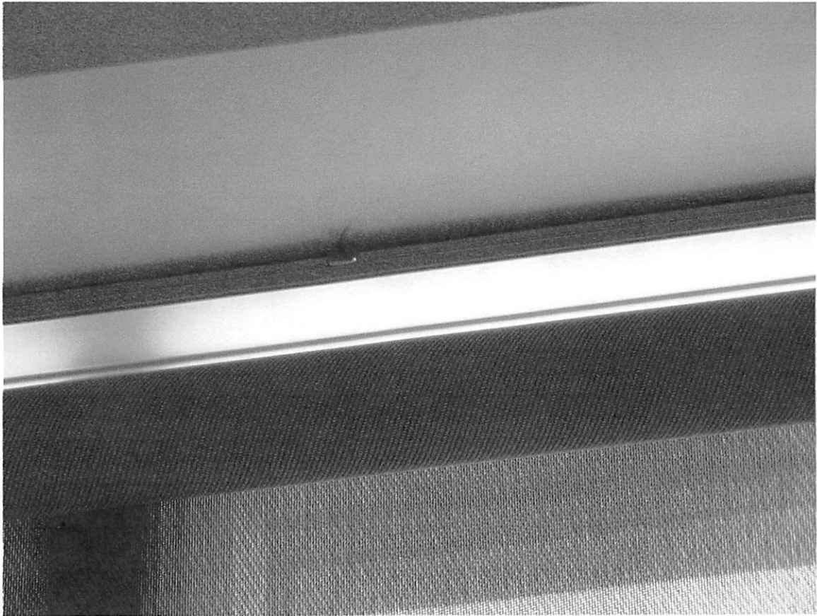
Sir John A. blind support screw in gyproc
